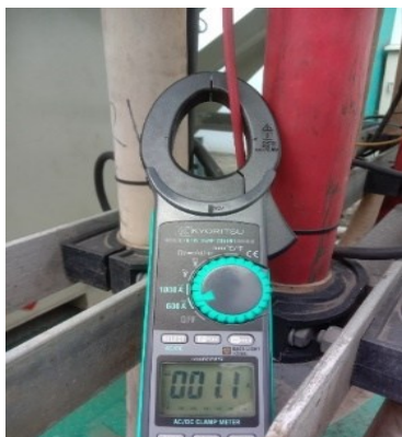
Figure 1. Leakage Current Measurement with Clamp Meter [24]
